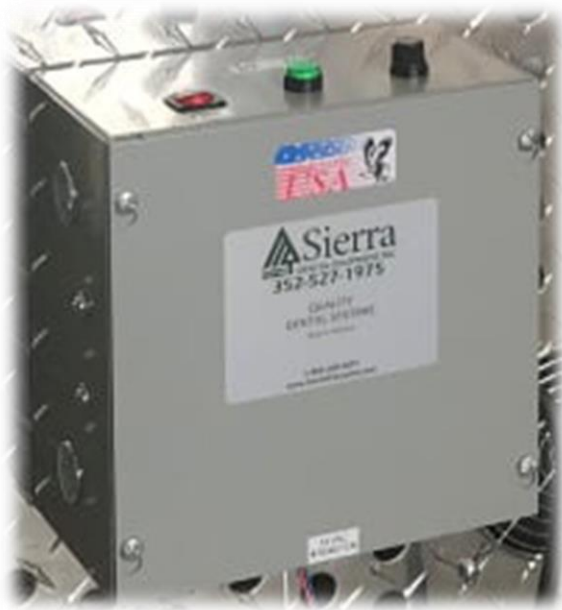
Low voltage control box
